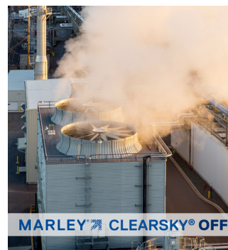
Patented ClearSky plume abatement system greatly reduces visible plume and conserves water.
