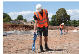
Safe underground infrastructure
